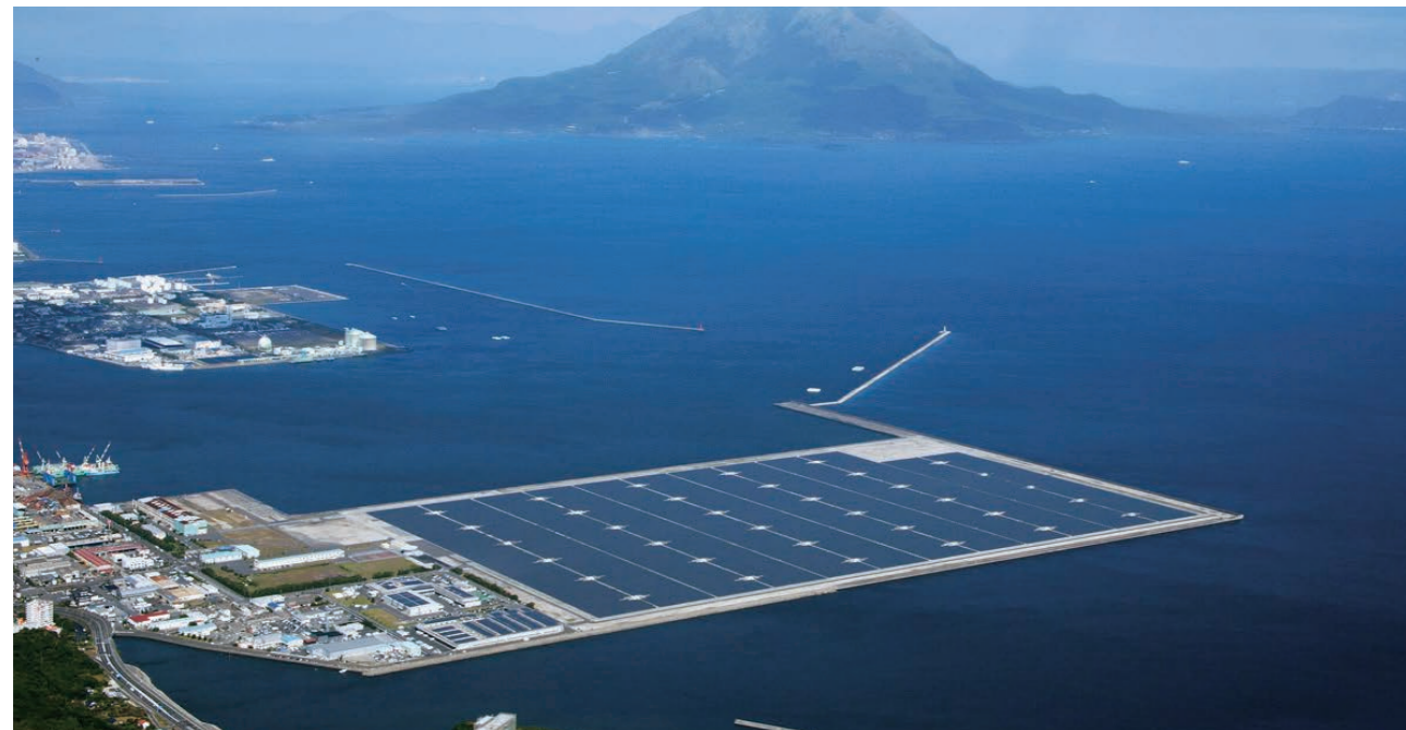
Large-scale megasolar project Kagoshima Nanatsujima Megasolar Power Plant
