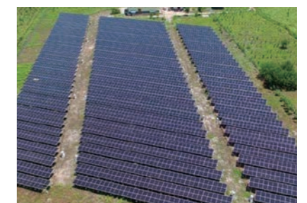
EMS demonstration facility (Sumba, Indonesia)
