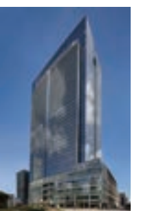
TOKYO MIDTOWN YAESU new construction work (electrical work)
