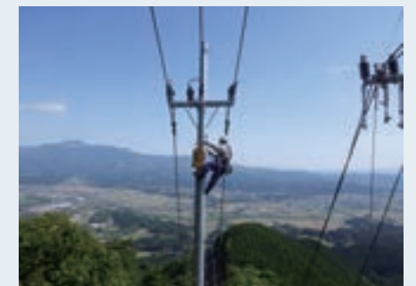
Interconnecting private line works associated with renewable energy generation plant construction
