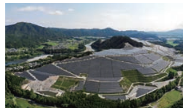
Miya River Watarai Solar Park
