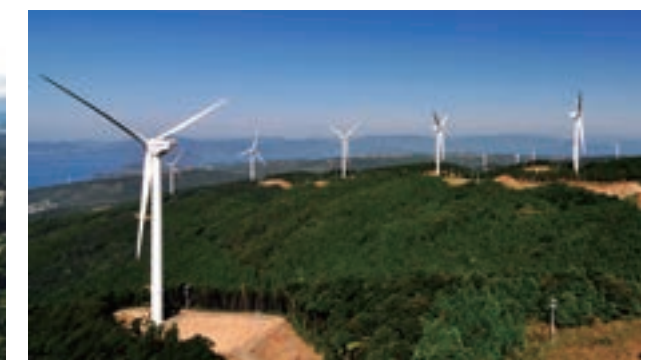
Kushima Wind Power Generation Plant
