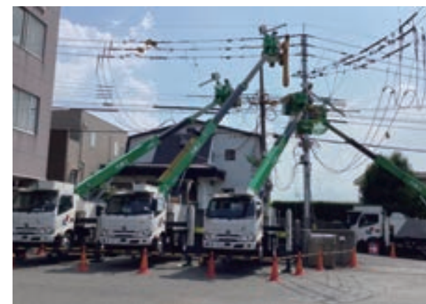
Contracted power distribution line work
