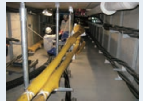
Underground distribution line work
